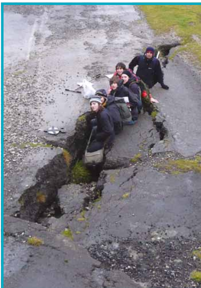
Students examine the effect of landslips in Natural Hazards
